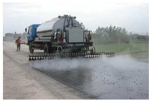
Automatic Bitumen Sprayer in Australia
